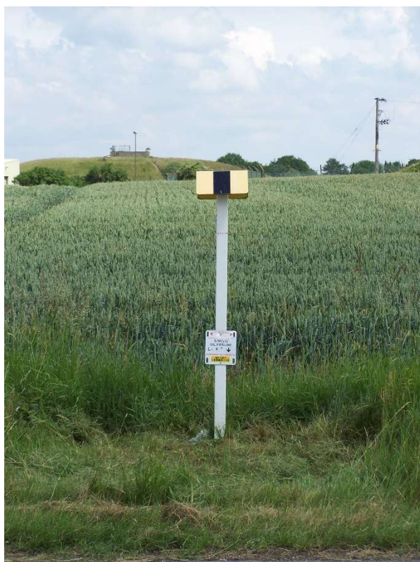
Figure 1.3: Post-World War 2 pipeline marker and marker plate, B1049 Woodwalton Lane (north), with fuel depot in background ©Sawtry History Society
