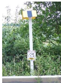
Figure 1.27: Pipeline marker and marker plate, Old Great North Road (east) ©Sawtry History Society
