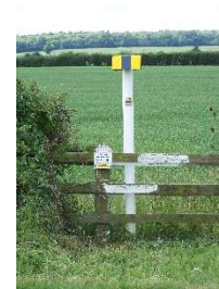
Figure 1.28: Pipeline marker and marker plate, B1049 Woodwalton Lane (south) ©Sawtry History Society
